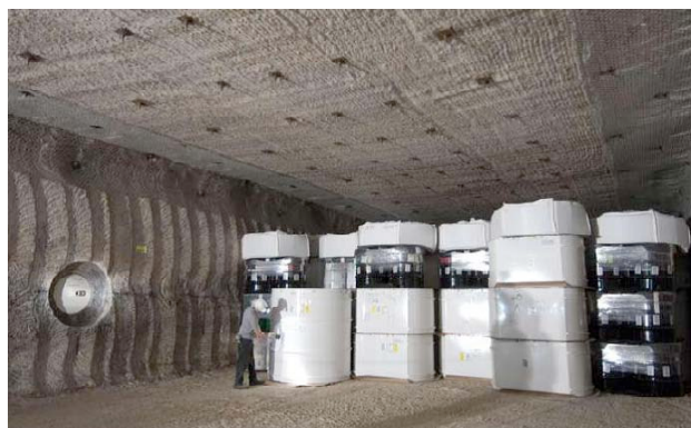
Fig. 5. Over 10,000 nuclear waste drums and standard waste boxes filling 1 of 56 rooms to be filled at WIPP over a 20-year period. Almost 25 rooms have been filled as of June 2008. Note the higher activity remote handled waste plunged into boreholes in the wall to the right and plugged.
